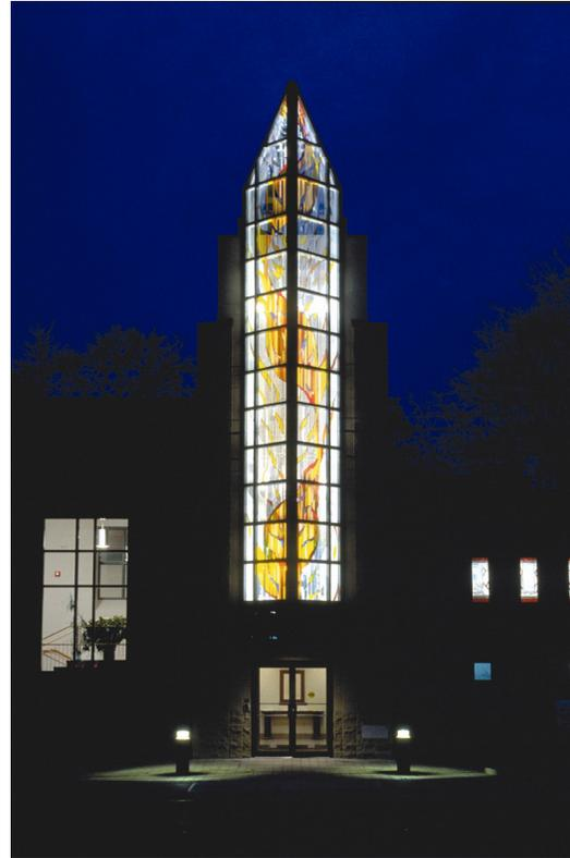
The photovoltaic array, embedded between two panes of glass, is composed of thin silicon and metal cells that convert sunlight into electricity. The energy collected will be used to illuminate the park at night with a changing color program inspired by the music of composer/violinist, Oliver Schroer. Containing 144 square feet of photovoltaic art glass, the installation also incorporates the Lord’s Prayer in Aramaic.
